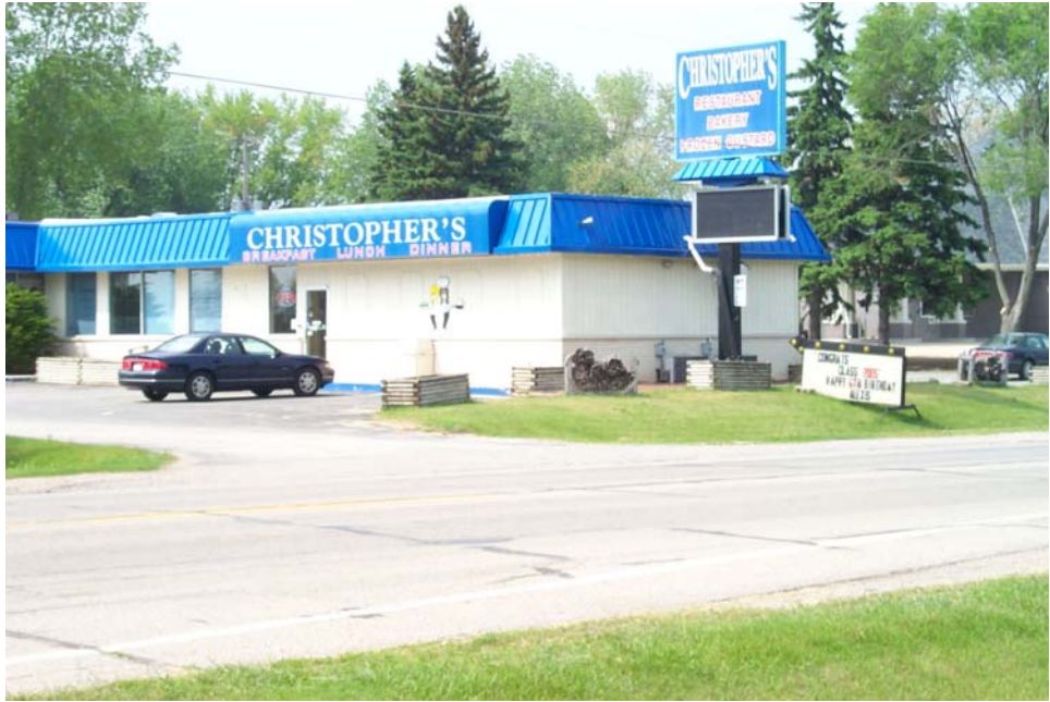
Very nice building, but portable sign detracts
