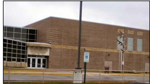
Photo: Example of a very nice investment in public infrastructure.
