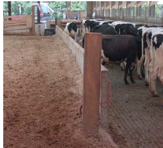
4 ft. high wall separates bedded pack and feed alley
