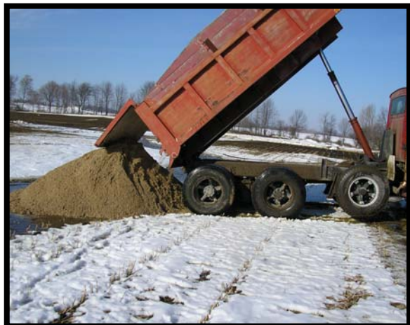
Create a dam to stop the flow of manure.
