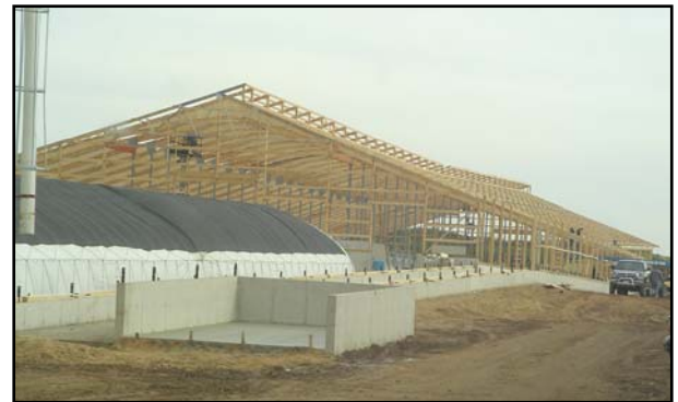
Construction of a 400 cow freestall barn at Egan's
