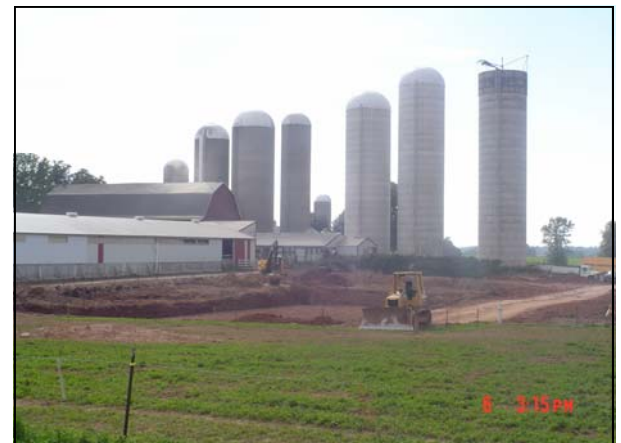
Excavation for total run-off containment manure storage system.
